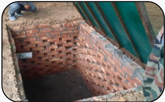
Sub-Surface Technique: Recharge Pit
