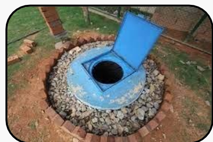
Use of drums in recharge pits
