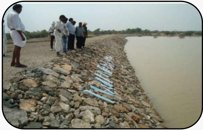
Surface Technique-Percolation Tank
